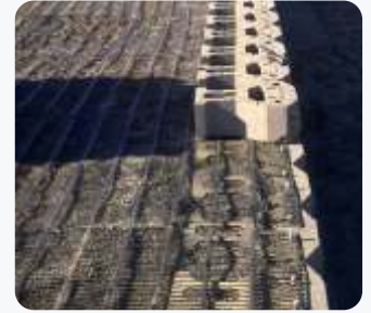
Reinforced earth wall
