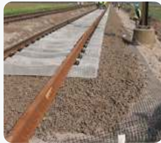
Existing Railways Tracks
