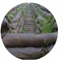
Ecobags in coffer dams
