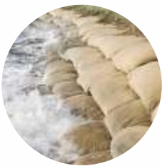
Coastal abrasion protection - ports and harbours, dams & levees
